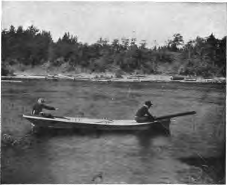
FIG. 53.—Wire and Boat Gaging Station.
